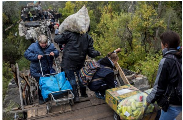
Stanytsia Luhanska broken section of the bridge before the repair, April 2019.
