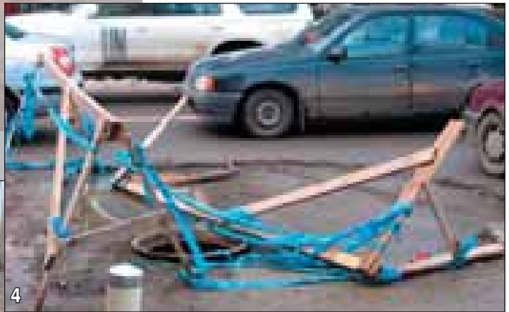
Photo 1, 2. Political party posters still hang on construction fences, leaving unresolved problems behind! Photo 3. This is one of the good examples that should be followed. Photo 4. Mind the hole! There is no proper hazard sign. Photo 5. Road repairs that started before the launch of the election campaign, still unfinished!
