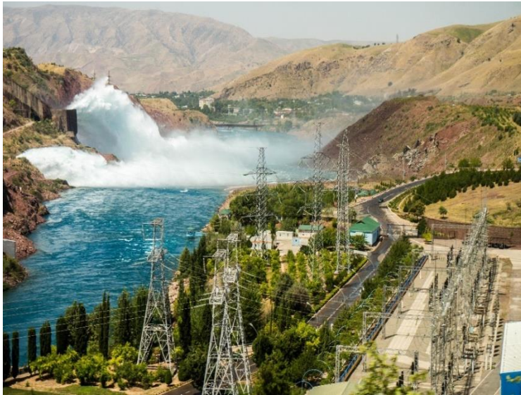
Photo 1. The Nurek HPP spillways and power substation. The HPP is responsible for over 75% of Tajikistan's energy supply (Photo: Ronan Shenhav, 2016)
