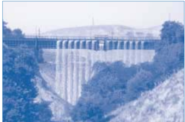
A water pipeline near Dushanbe.
