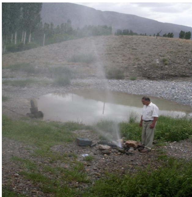
Photo 3. Breakdown in “Vorukh-Shurab” Water Pipeline Route
