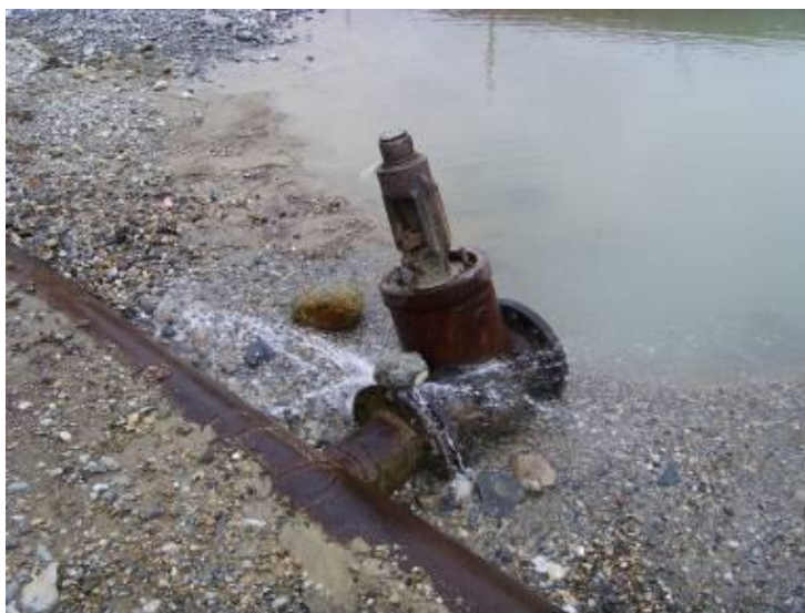
Picture 11: Section in critical condition on water pipeline route between Points 3 and 4
