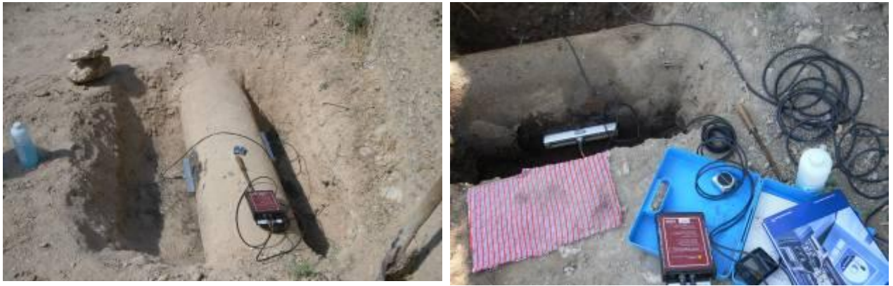
Picture 9,10. Preparation of Ultrasonic Water Flow Meter at the Measuring Point
