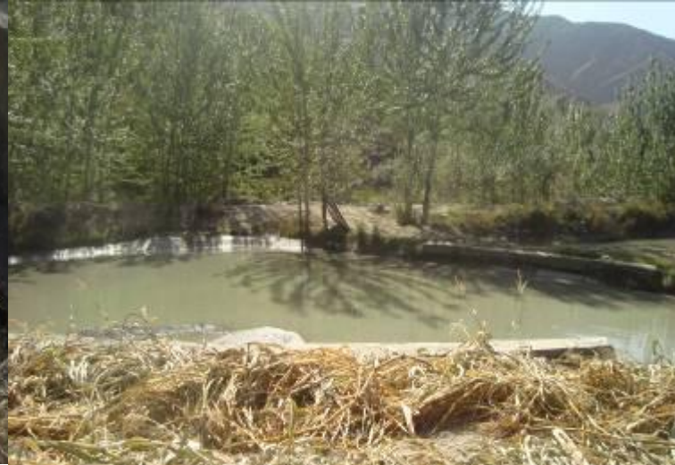
Picture 14. View of the first settling
