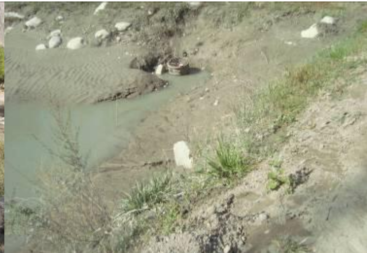
Picture 16. Typical silting of settling
