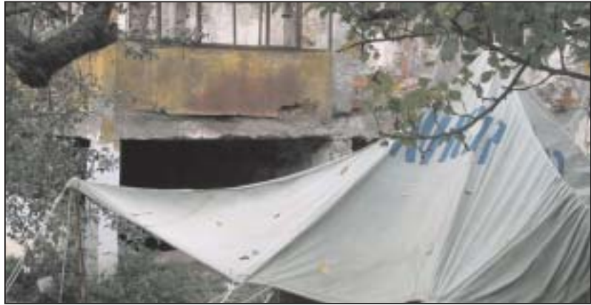
Returnee's house waiting to be restored
