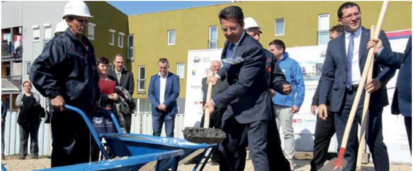
The Head of the OSCE Mission to Serbia, Ambassador Andrea Orizio, at a groundbreaking ceremony for the construction of 40 apartments in Sremska Mitrovica, held as a part of the implementation of the Regional Housing Programme Sub-project 2 in Serbia, Sremska Mitrovica, 17 March 2017. (OSCE/Milan Obradovic)
