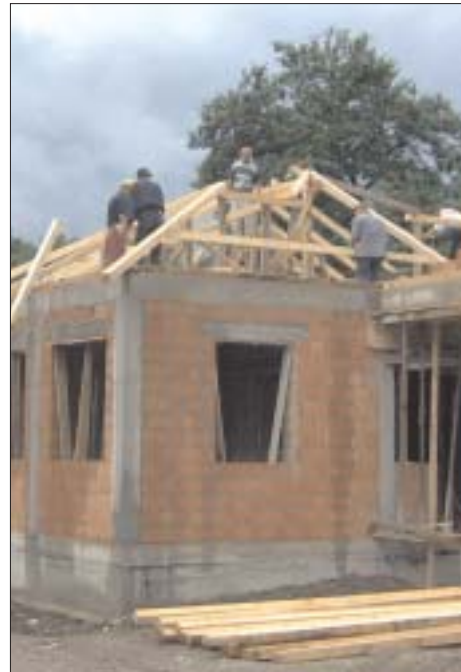
Workers building the roof of the Ambulanta
