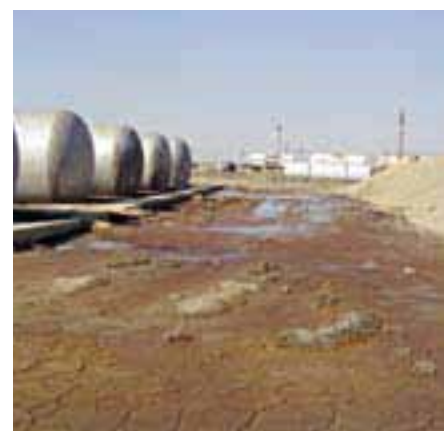
Site of leaking Melange containers, Azerbaijan
