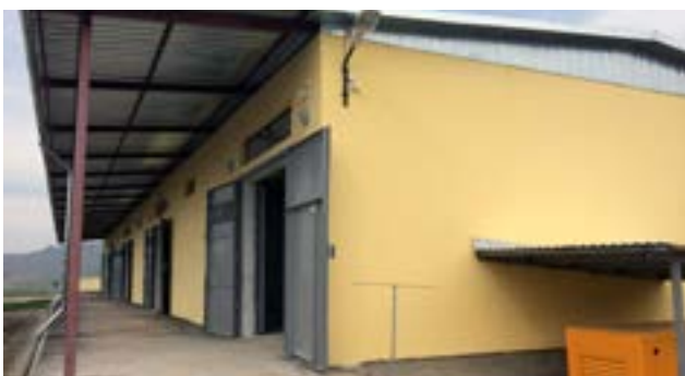
The OSCE Centre in Bishkek's ongoing programme on small arms and light weapons and conventional ammunition supported the reconstruction of warehouses for the Kyrgyz Armed Forces and constructed a new warehouse at a military unit in the village of Koi-Tash, 20 km from Bishkek. (OSCE/Vasilina Brazhko)
